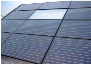
Rooflights & Solar PV Tiles
